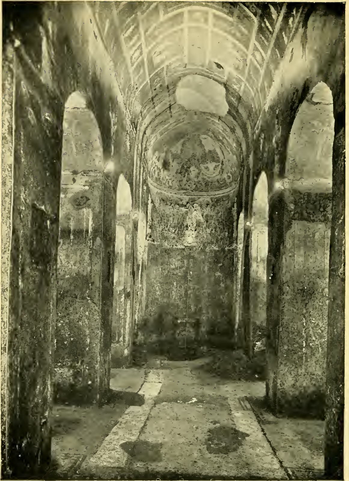
Fig. 43. INTERIOR OF SUBTERRANEAN BASILICA Near the Porta Maggiore, Rome. 1st cent. A. D.
